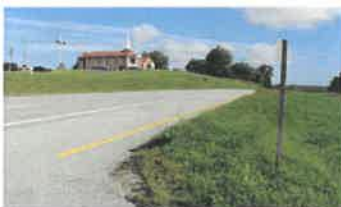
Looking north at southbound lanes from median
