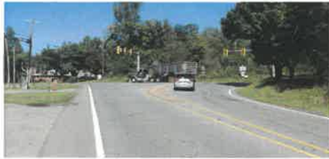
Westbound approaching Amherst Highway
