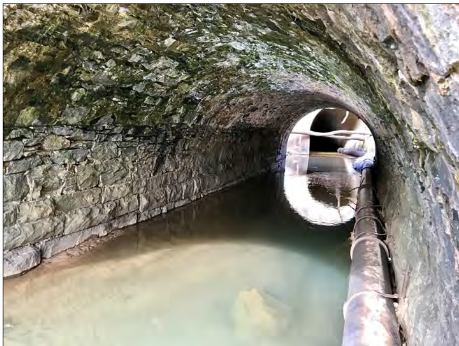
This older stone culvert carries what is now Macon Street across the South Fork. The newer concrete culvert carrying the current NS railroad can be seen in the distance. A town sewer pipe currently utilizes the passage.
