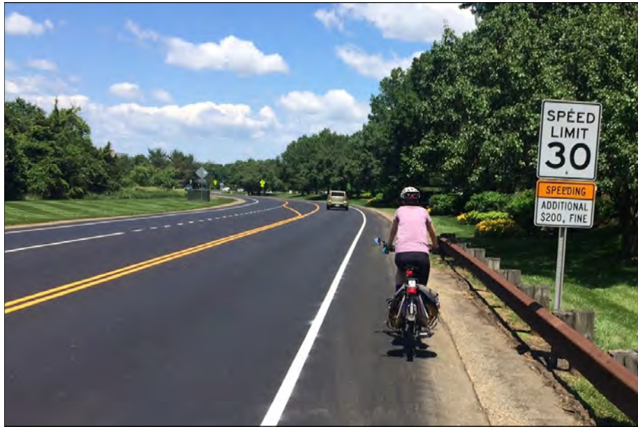
An example of a paved shoulder.
